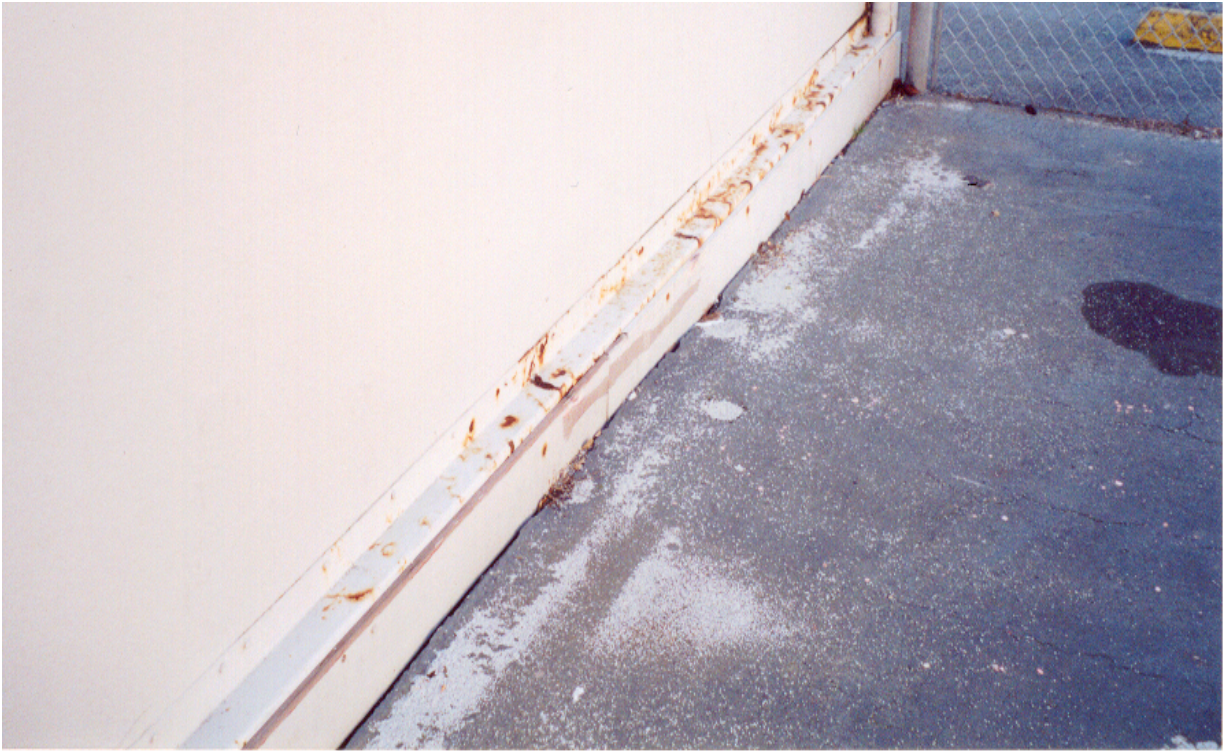
Figure 15: Rust at Base Frame of Portable Unit
