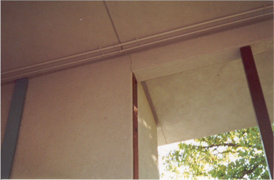
Figure 12: Cracks at Rear Side of Entrance Canopy at Building
