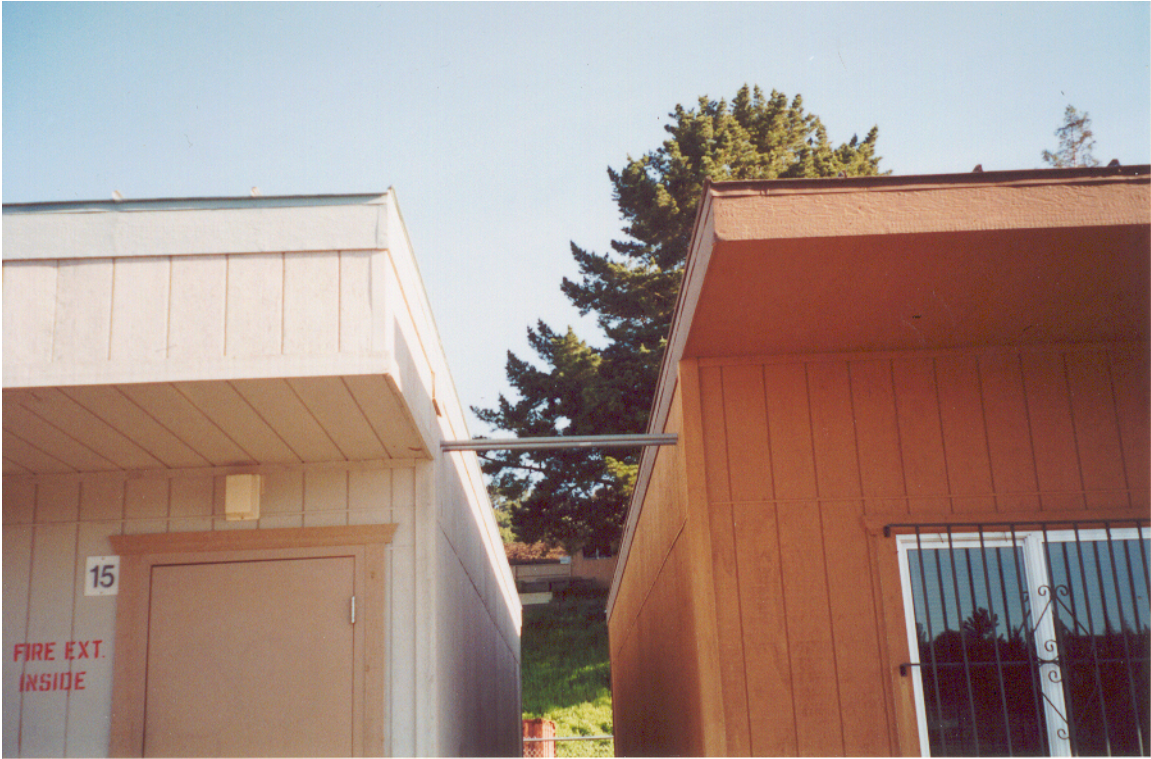
Figure 16: Conduit Running between Portables
