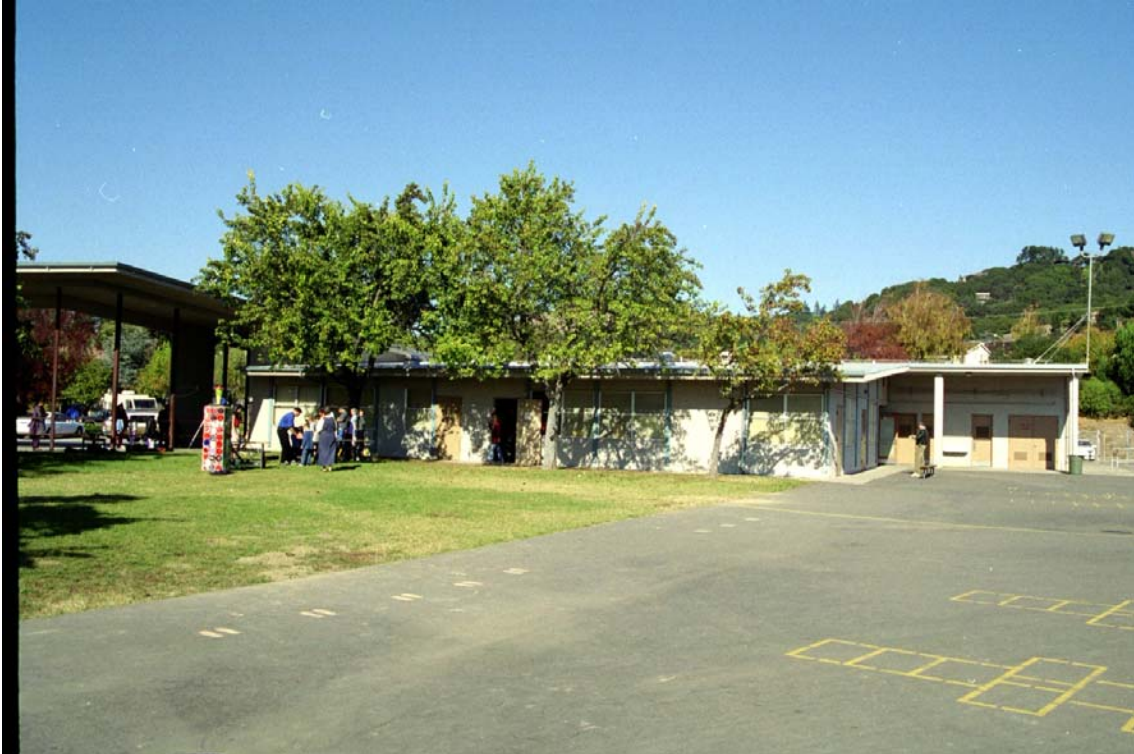
Figure 3: Wing A Classrooms (front)
