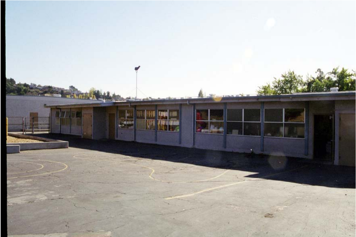
Figure 4: Wing A Classrooms (rear)
