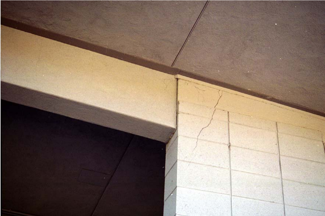
Figure 9: Cracking at Entrance Canopy
