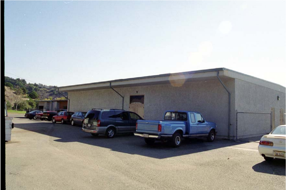
Figure 8: Multi-Purpose Building (rear)
