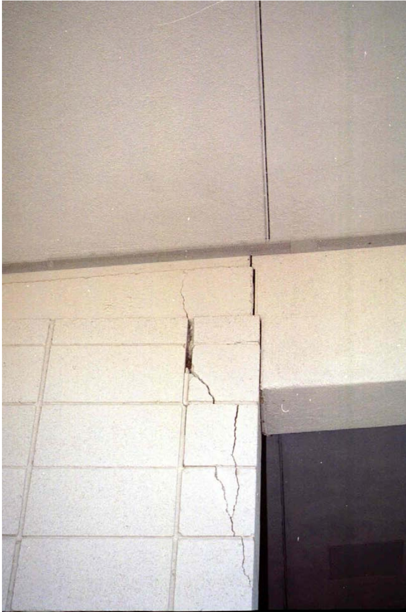
Figure 10: Cracking at Entrance Canopy
