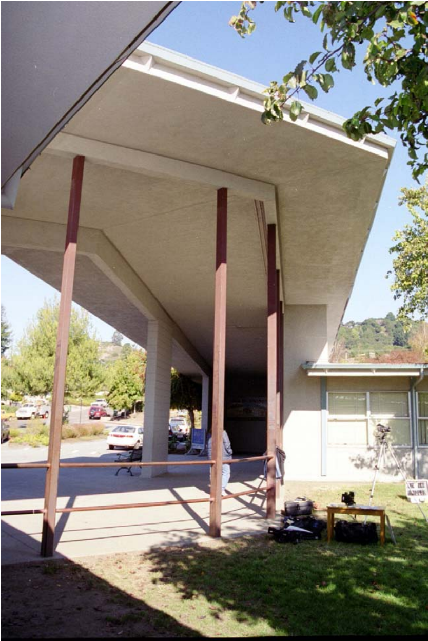
Figure 11: Columns at Entrance Canopy
